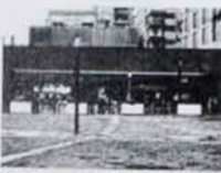
Woolwich N51.5200° E008°00'55.60" Underground
